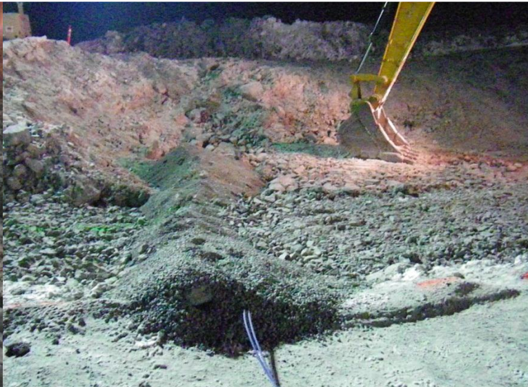
Photo 9: Thermistor cables at 0+60 bedded in 3/4" material.
