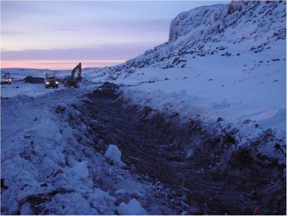
Photo 7: East end of the Doris North Diversion Berm key-trench after cleaning was performed by excavator.
