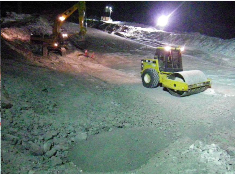
Photo 10: Compactor running on transition material placed in 'hole' around thermistor cables at 0+60. Looking down at the 'hole'.
