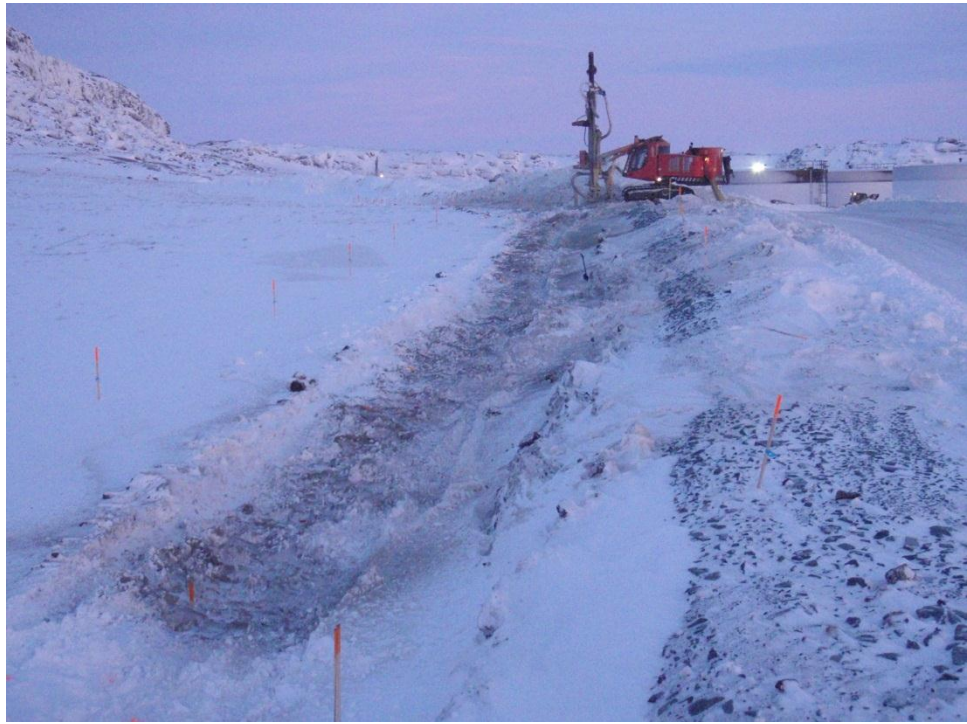
Photo 6: Westarc drill continued drilling along the Doris North Diversion Berm key-trench.
